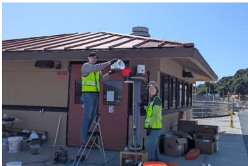
Secondary Clarifier Stress Testing
